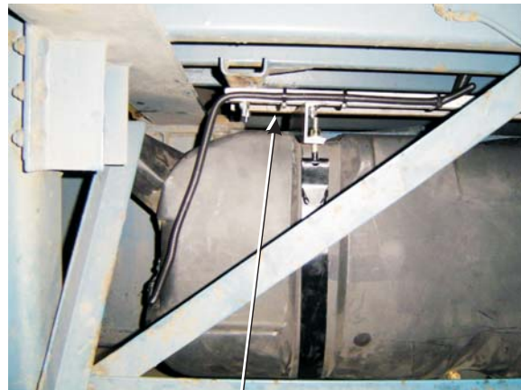
Route harness along the support and bandwrap
